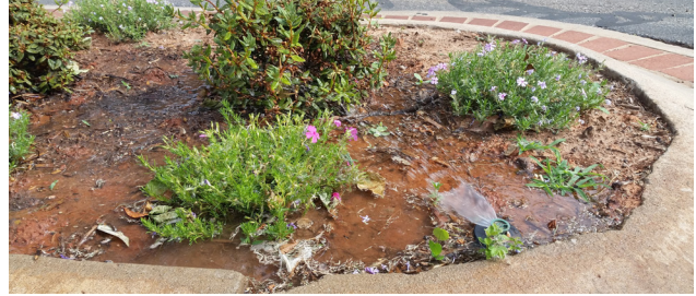
Figure 6. Sprinkler head stuck and failing to fully pop up above the ground.
